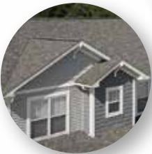
Roofing and Ventilation
